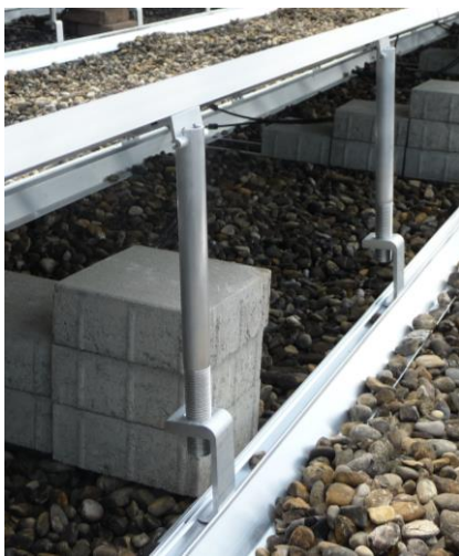
Figure 31 Height adjustable module support
