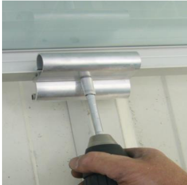
Figure 63 Installation of front module bracket set
