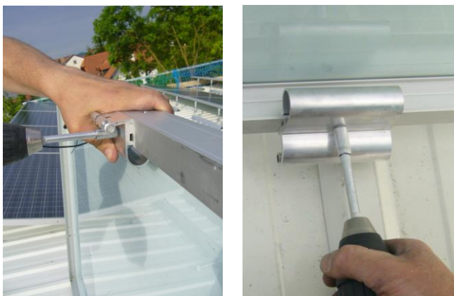
Figure 29 Installation of the Module bracket set at the rear (left) and front (right)
