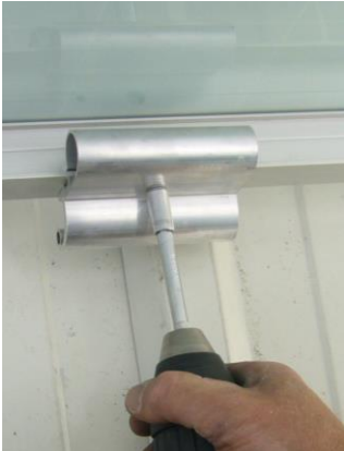
Figure 45 Installation of module bracket set (front)
