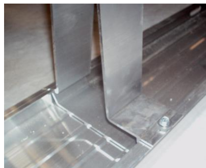
Figure 58 Support set in base trough
